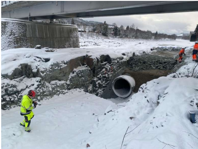
Figur 10: Masser rundt kulvert basal 1600 mm
