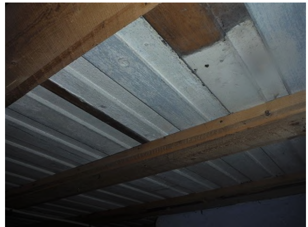
Figur 25: Gammelt stubbloftsgulv
